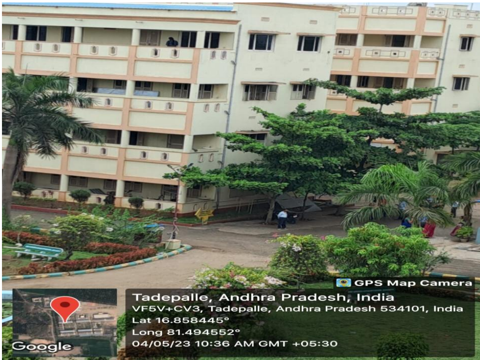
Fig. Rain water collection from roof top
