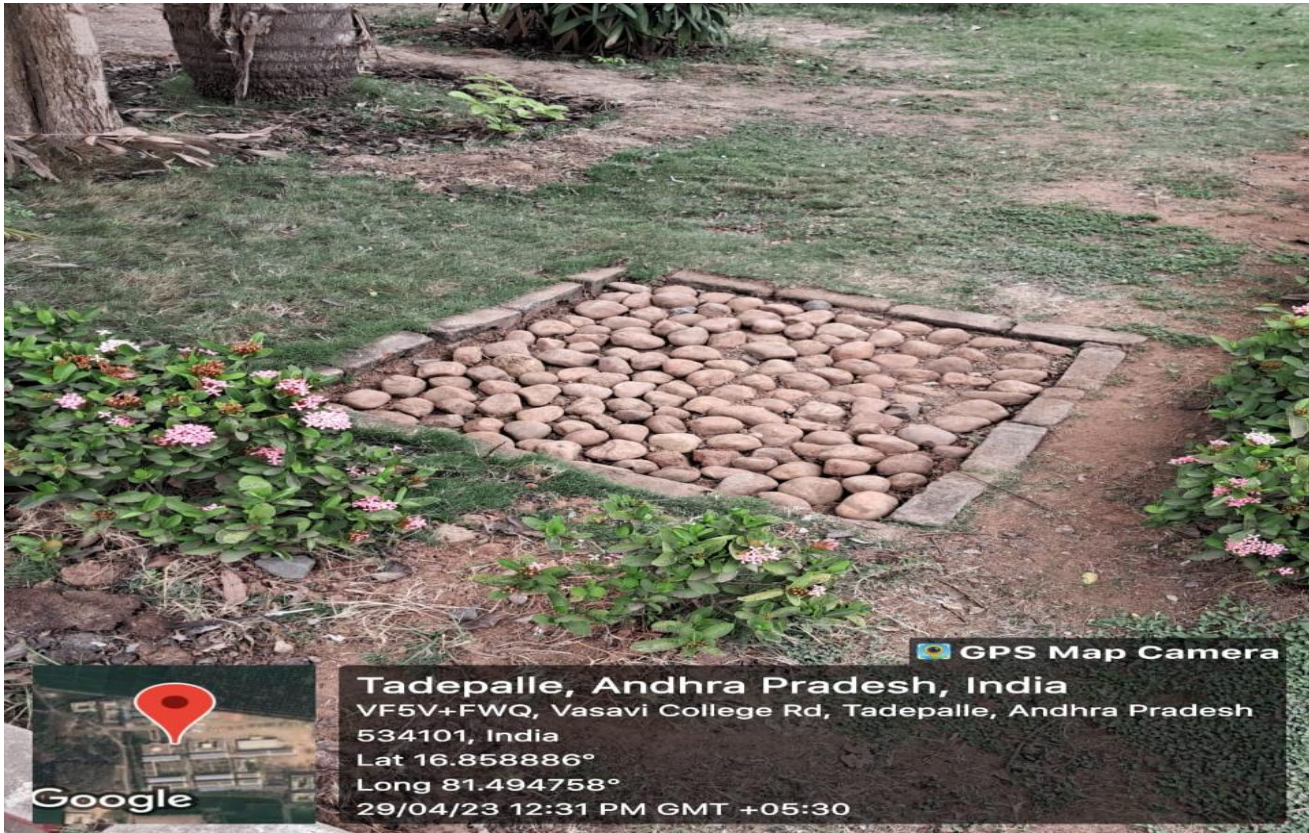
Fig. Borewell/Ground water recharging through Rain water harvesting
